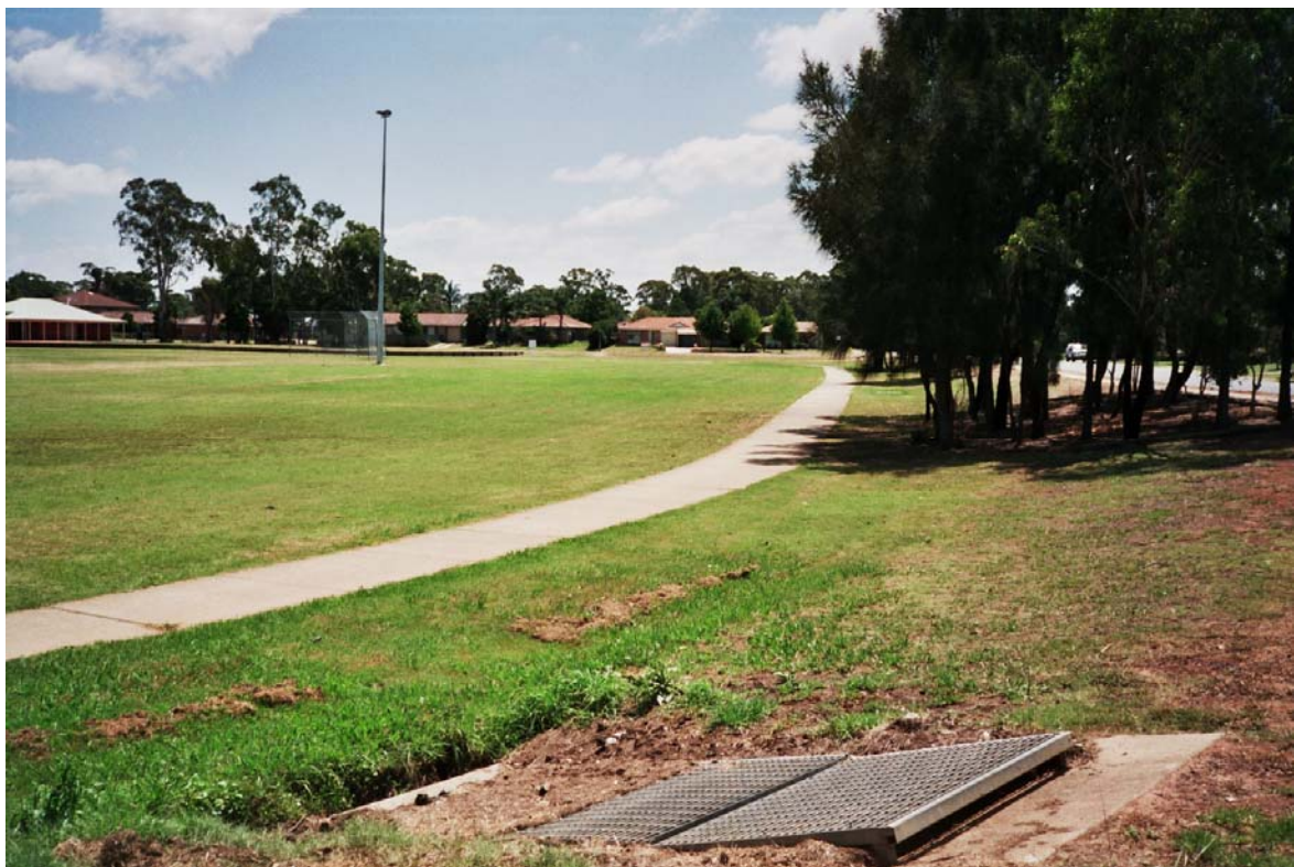
Photograph No. 1: View of Colonial Reserve basin from near BP10 in Guardian Crescent. Basin outlet pit is in foreground.
